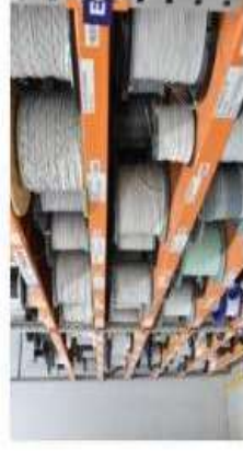
Facility - Cable bobbins in rack
